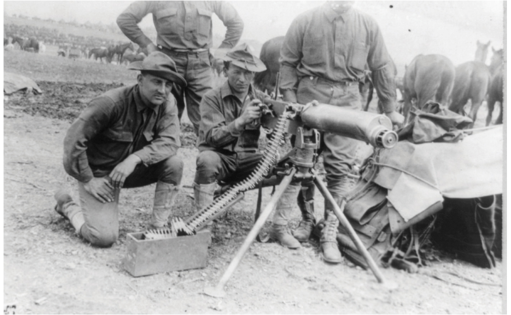
This crew of four men armed with a Maxim gun could wipe out an entire regiment in seconds. Early machine guns required a crew to feed ammunition and circulate water through the weapon to prevent it from overheating.
