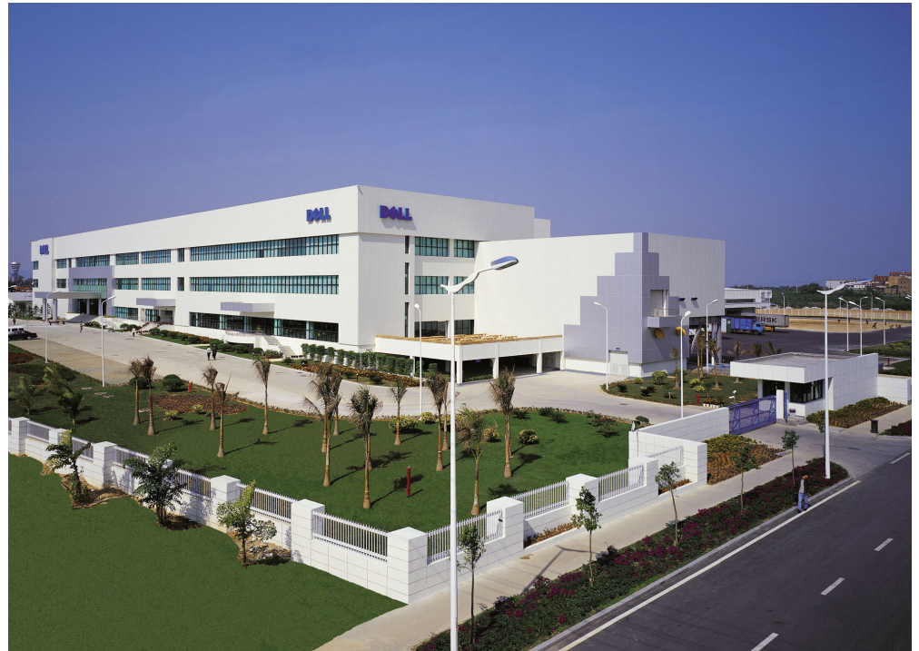
Figure 10.5 Dell's Local Operations in Xiamen, China
