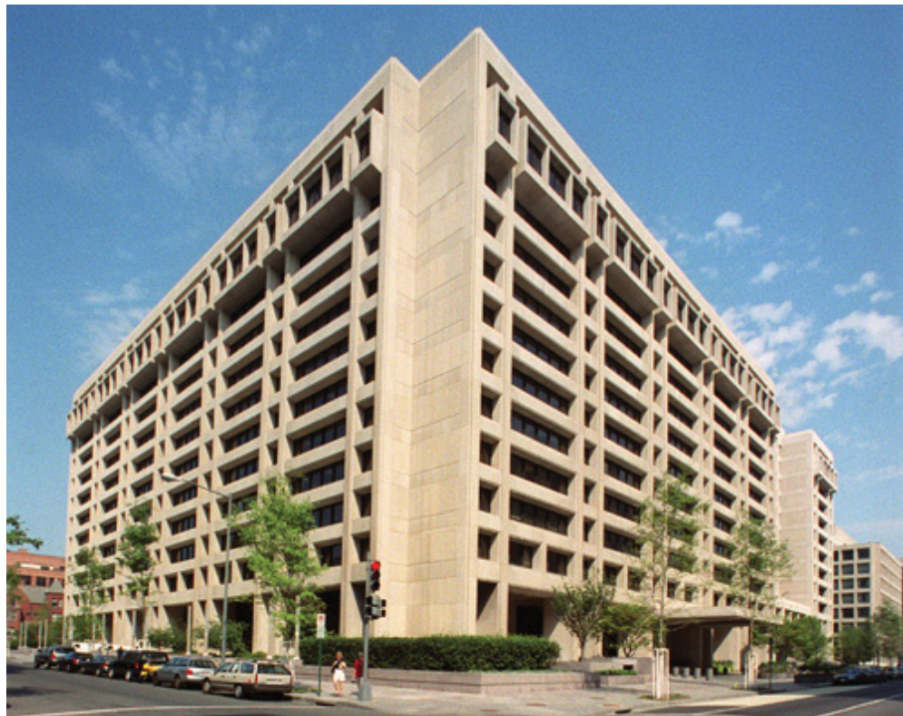
Figure 6.1 IMF Headquarters in Washington, DC
