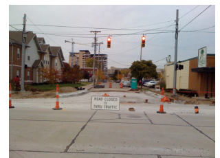
Figure 7.1 A Typical Construction Site
