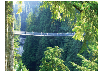
Figure 10.5 Capilano River Bridge
